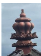
Fig 3. Use of Fiberglass Material on the Badung Regency Government Center Building. Source: Author
