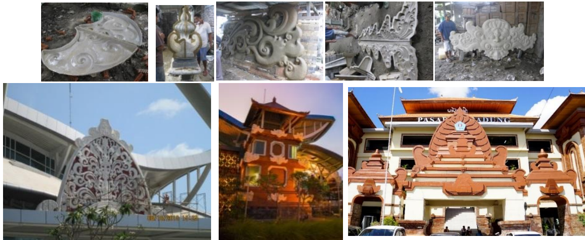
Fig 6. Use of Precast Concrete Ornaments at Ngurah Rai International Airport
